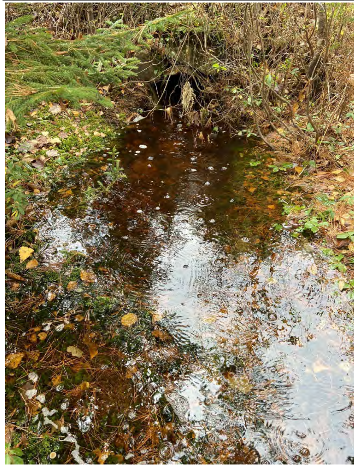
Photo 1: Flow at crossing through culvert after heavy rainfall event
