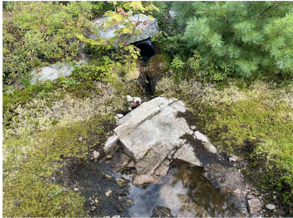
Photo 1: Culvert looking downstream of crossing location.
