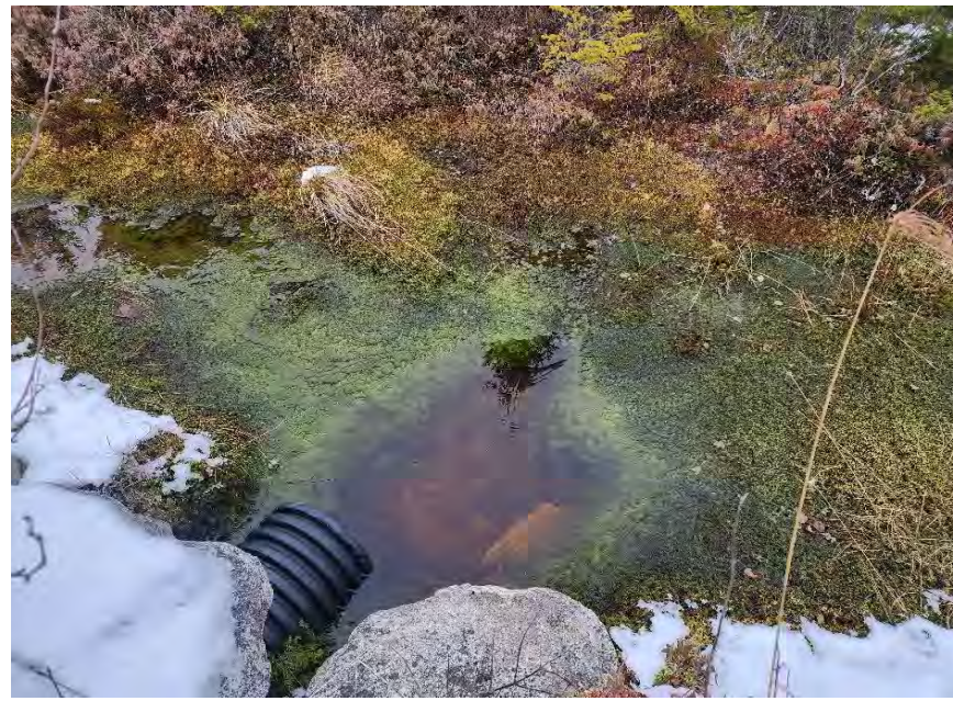
Photo 1: Culvert upstream at Crossing
