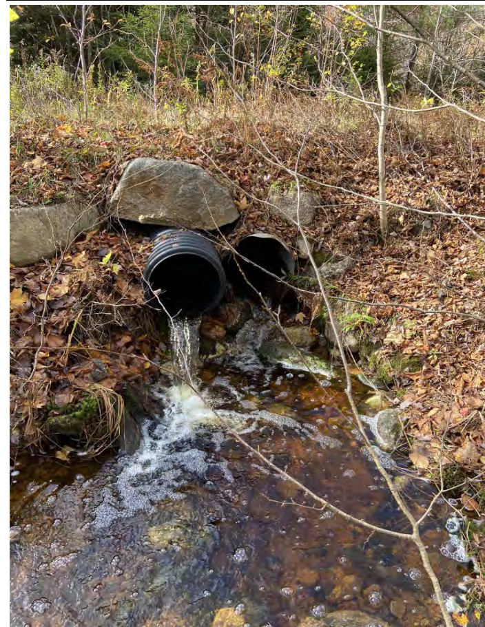
Photo 1: Upstream at crossing
