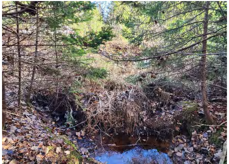
Photo 2: Downstream at Crossing, completely covered culvert
