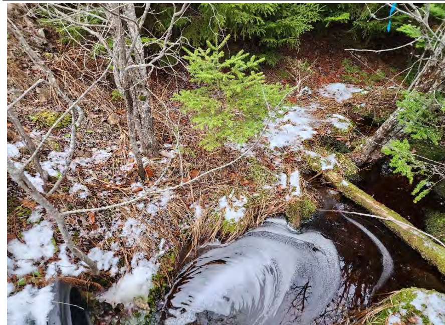
Photo 1: Upstream at Crossing with culvert
