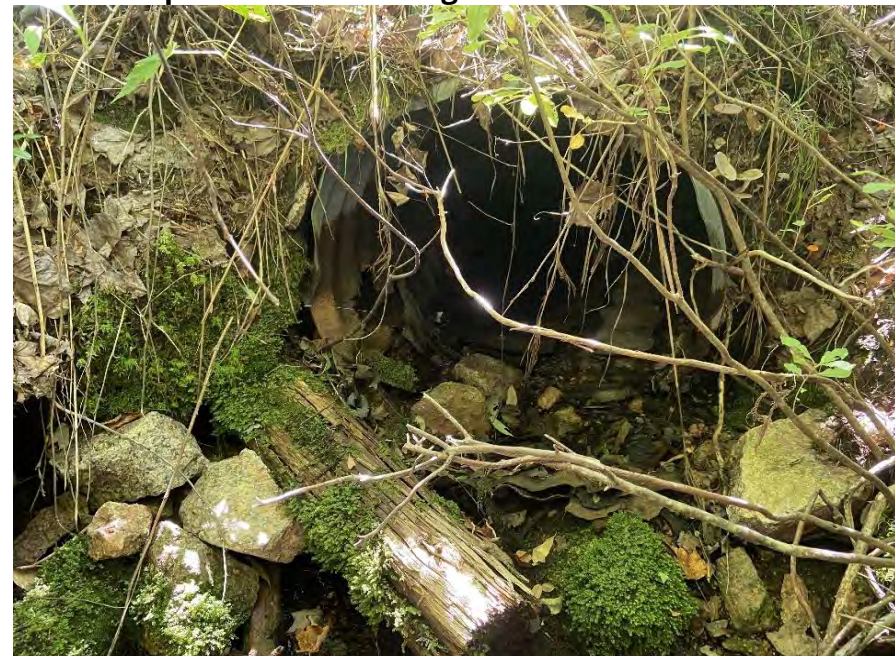
Photo 2: U/S Culvert showing low water level
