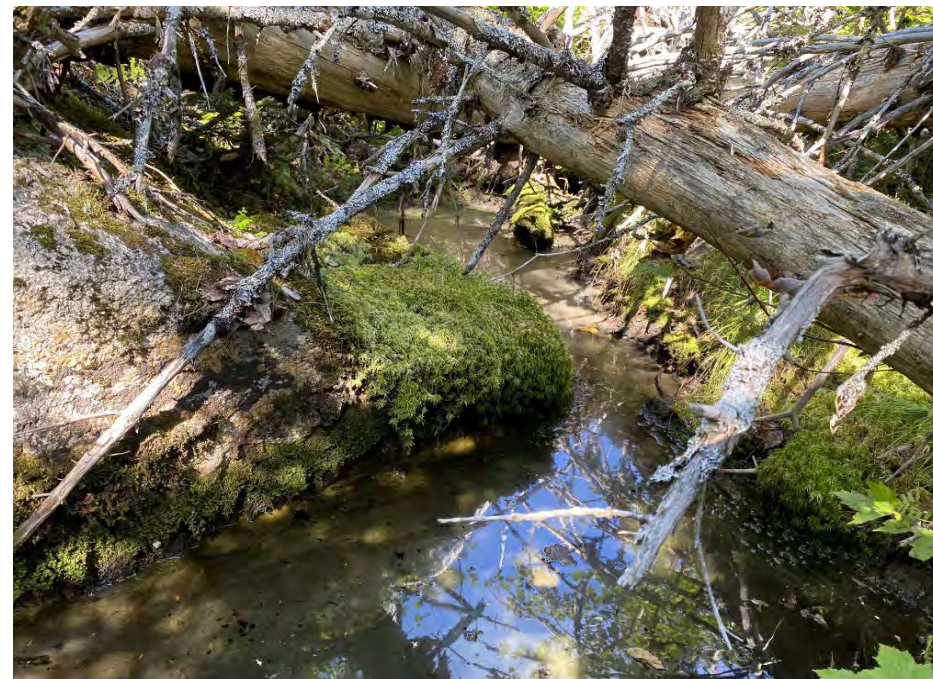
Photo 2: Downstream at assumed crossing
