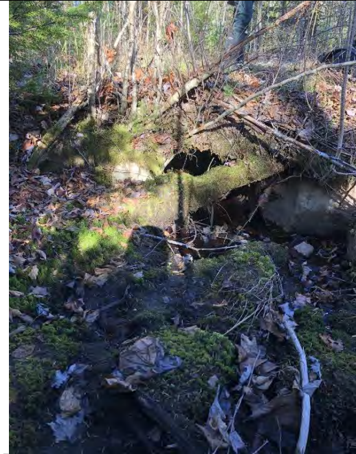
Photo 1: Upstream at Crossing
