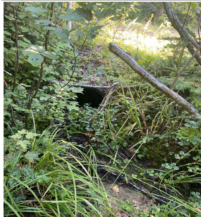
Photo 1: Culvert at crossing
