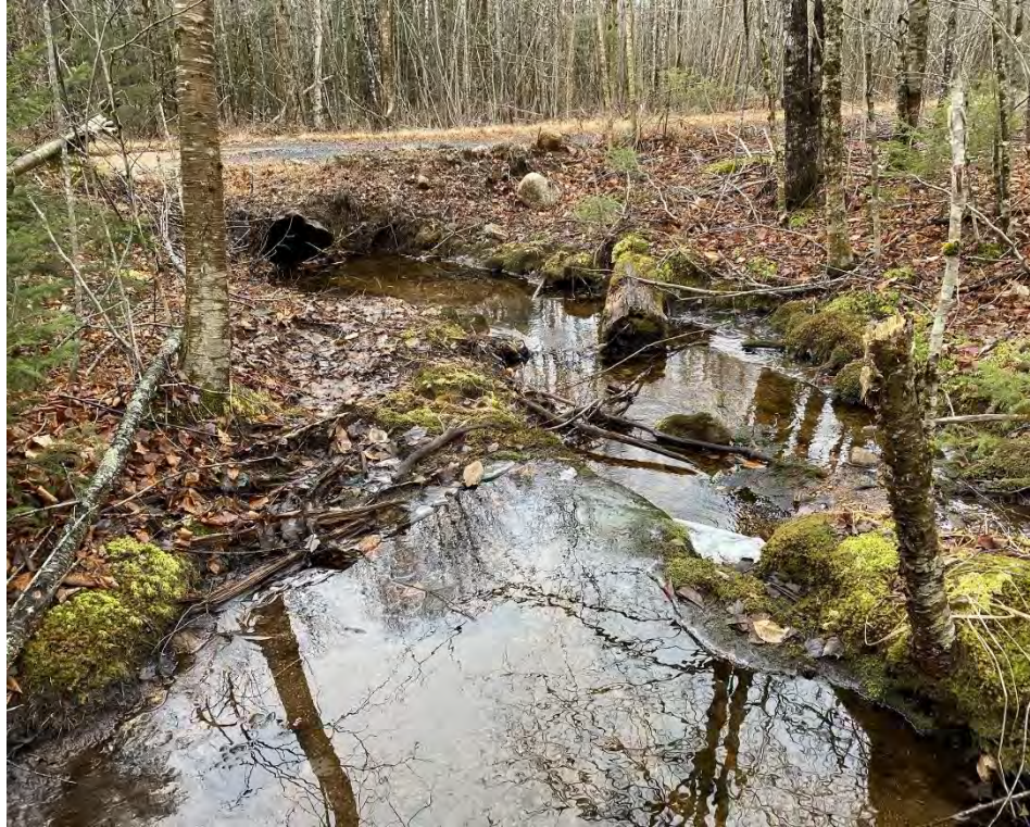
Photo 3-10 Looking downstream at crossing location.
