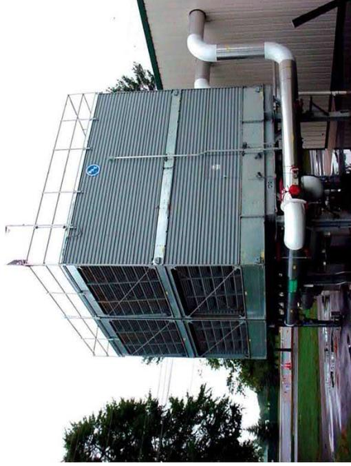
Cooling towers are required to reduce high summer water flows. This will in turn reduce the total effluent flow.
