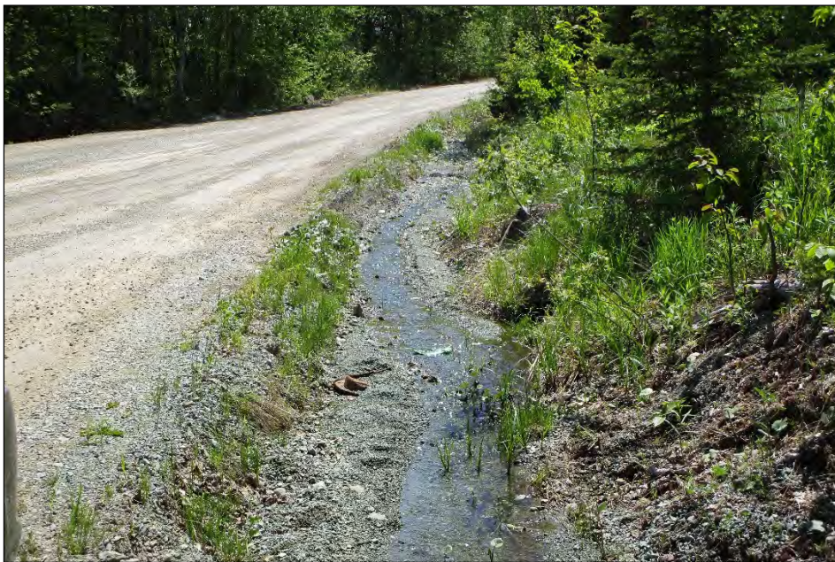
Figure 13. Seepage flow from quarry base along access road at weigh scale, June 8, 2017.
