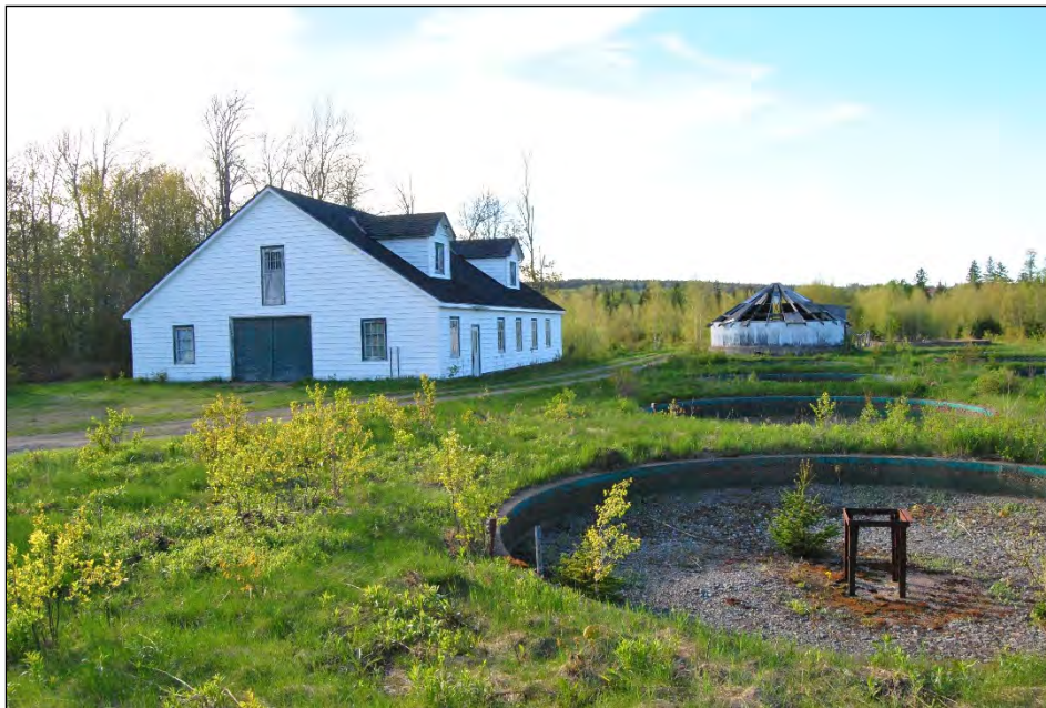
Figure 31 Abandoned federal government fish hatchery on Wentworth-Collingwood Road at Jackson. Hatchery was divested by Fisheries and Oceans Canada in the late 1990s and subsequently closed.
