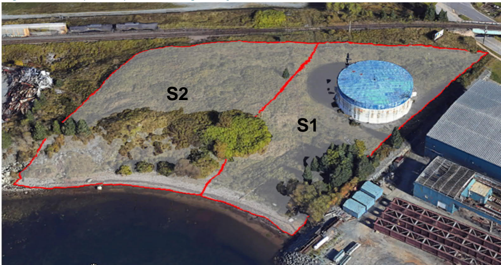
Figure A-1: Liquid Asphalt Storage Project Area Subcatchments
