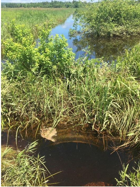
Photo 5: Culvert beneath D2 trail crossing (July 3, 2019).
