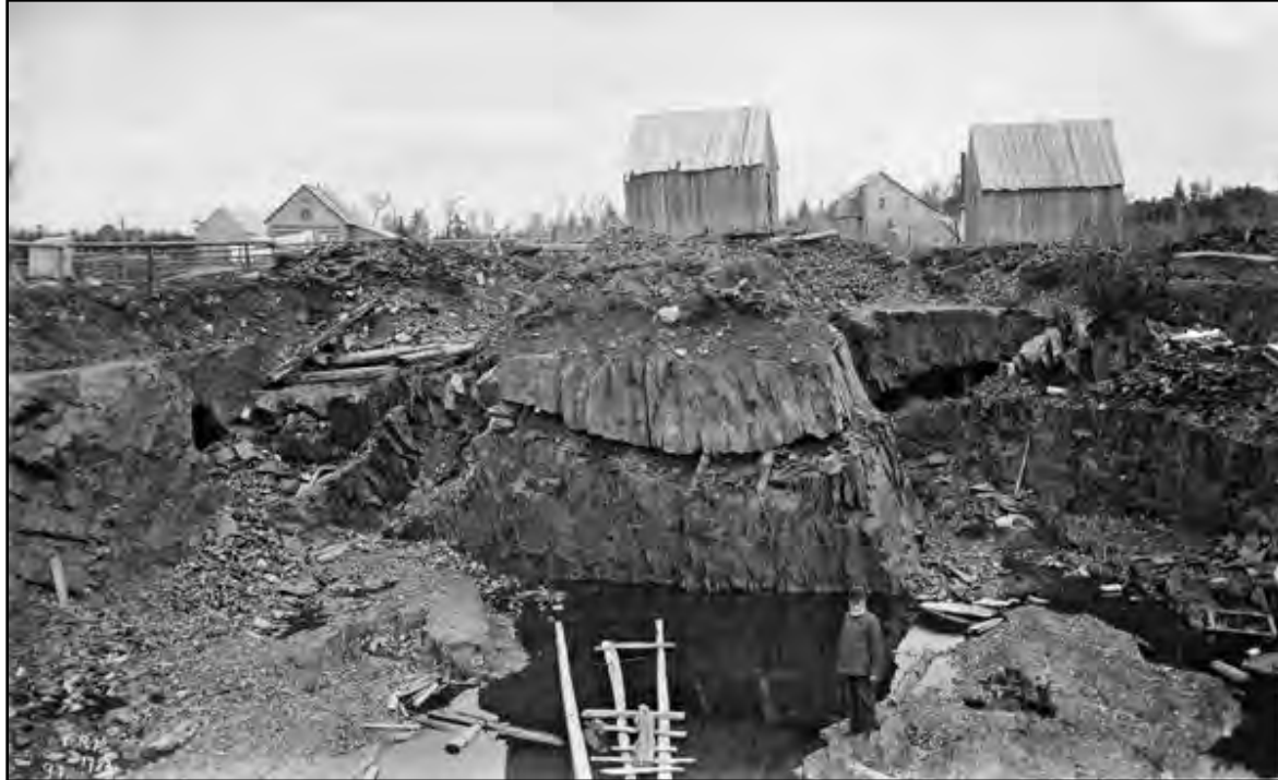
Plate 12: Taylor lead on the crown of the anticline, Moose River Gold District, 1897 (Faribault)
