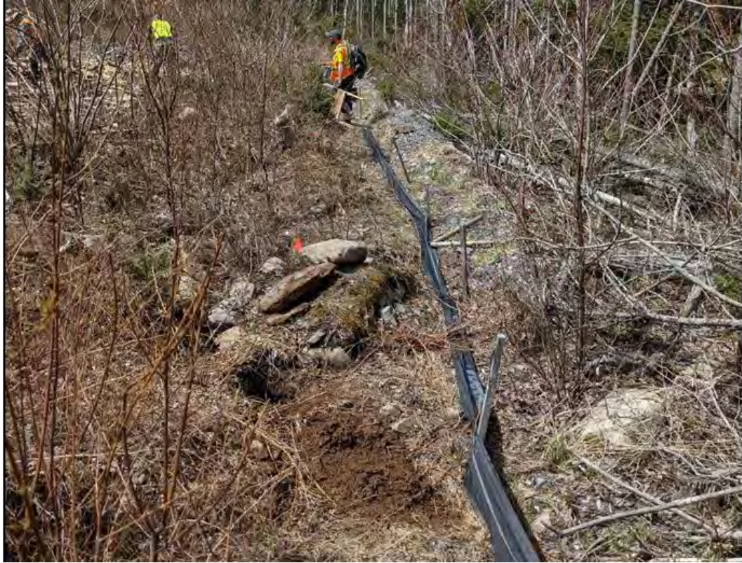
Plate 15: Silt fencing installed within mechanically excavated trench; facing northwest. 28 April 2021
