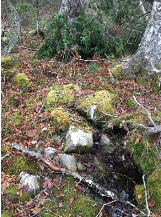
Photo 5. Drainage feature along WC1 (November 2019)
