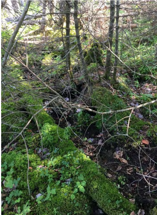
Photo 1. Drainage feature along WC1 (July 2019)
