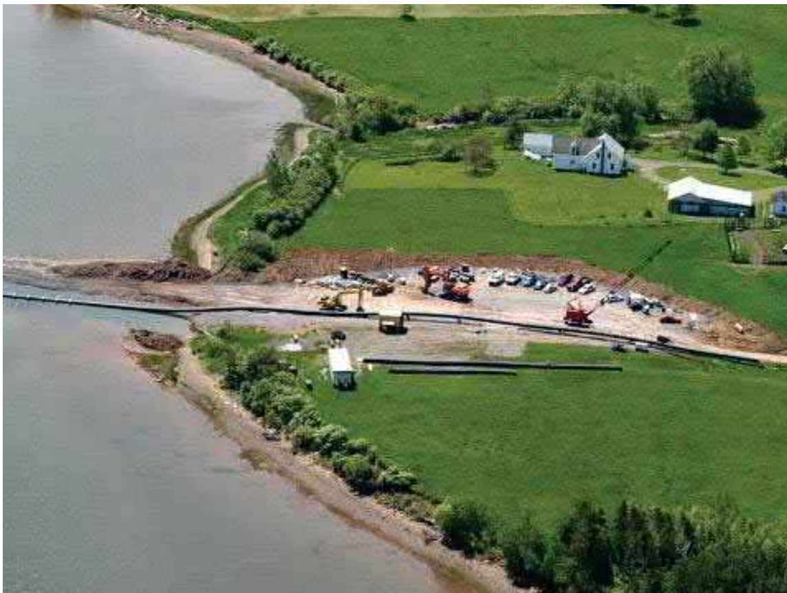
Figure 4-5 East River Shore Construction of Mill's Effluent Pipeline Replacement in 2009
