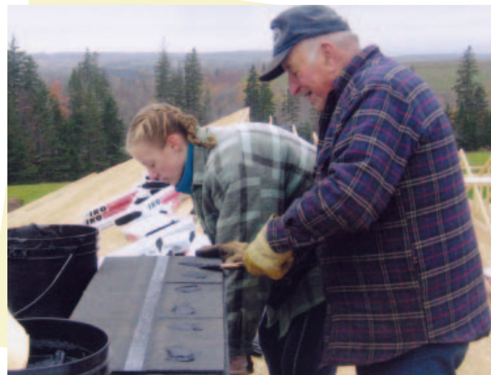
Photo above: Volunteers of all ages lend a hand in creating affordable rental housing for seniors in St. Andrews, Antigonish County.
