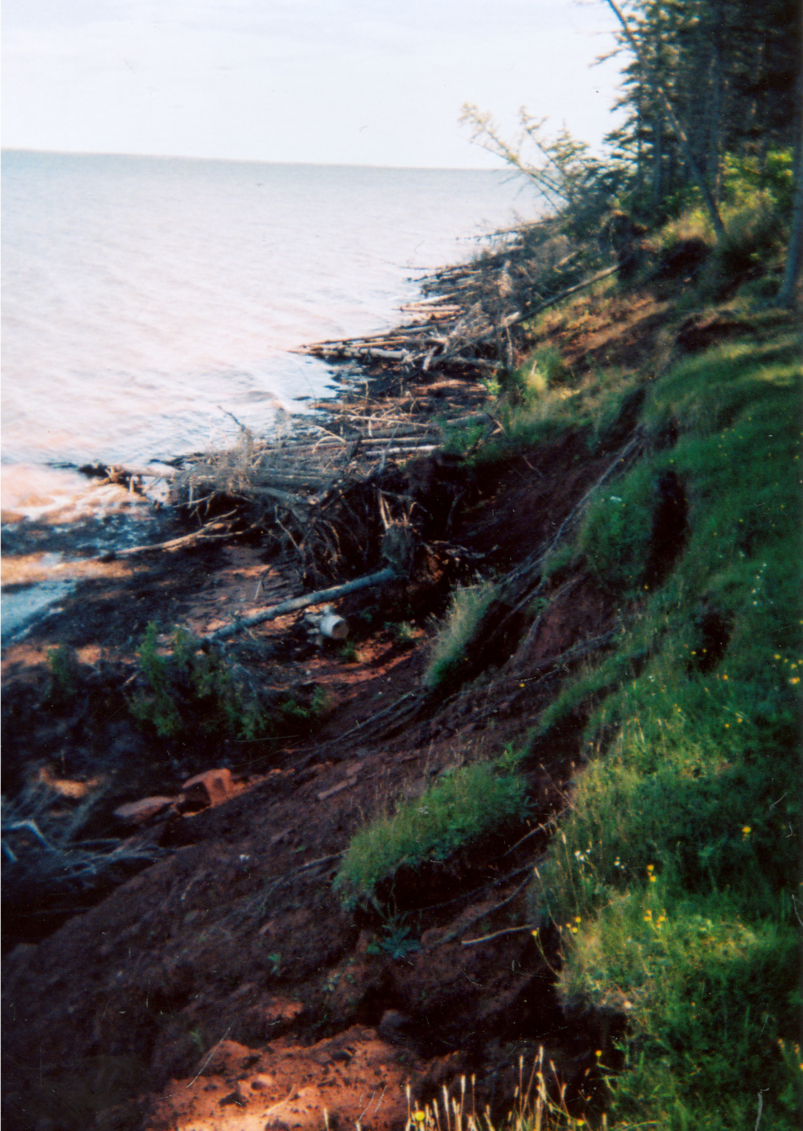
Figure 9. Erosion of Eatonville Till along the bank of a heavily wooded shorefront property. Trees are undercut and collapse outward onto the beach, suggesting that the shallow spreading root systems of the softwoods are having little effect in reducing the rate of erosion.
