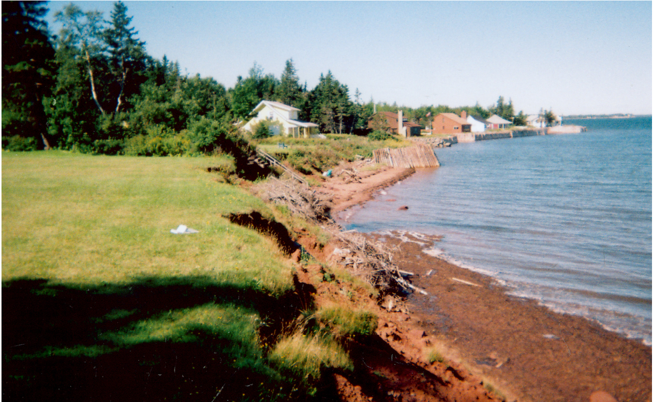
Figure 8. Extensive erosion of Eatonville Till along the bank of a shore front property. The owner has chosen not to armour the shore face; his cottage is located well inland from the bank edge. Note the armouring in the background and the lack of exposed beach at near high tide.
