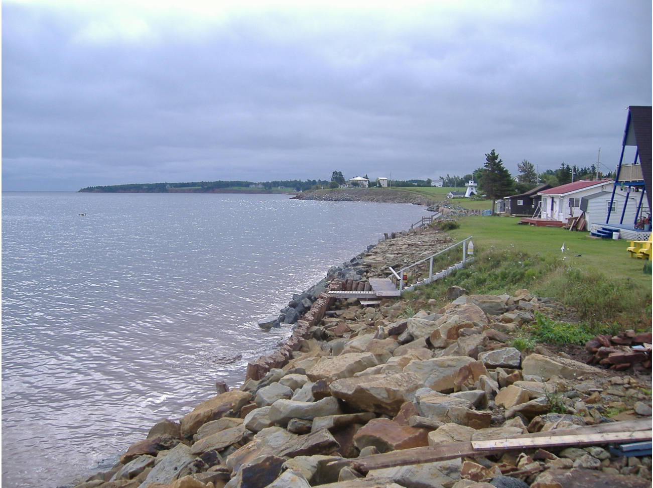
Figure 6. The shore face has been widely hardened in the study area using a combination of wood retaining walls and more recent armour stone.
