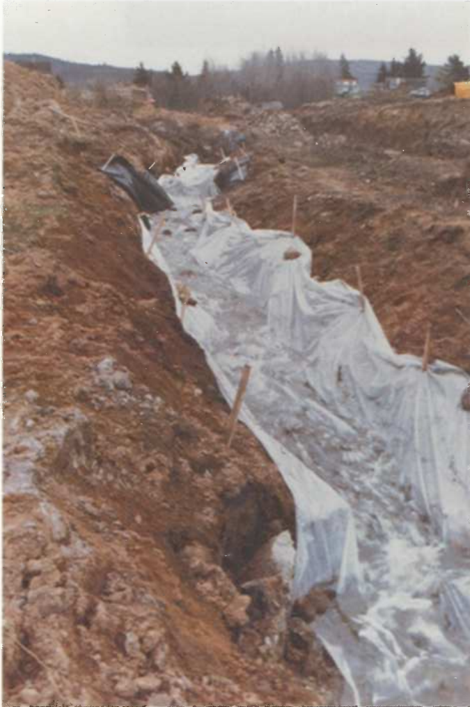
Polyethylene liner used to protect a temporary diversion ditch.
