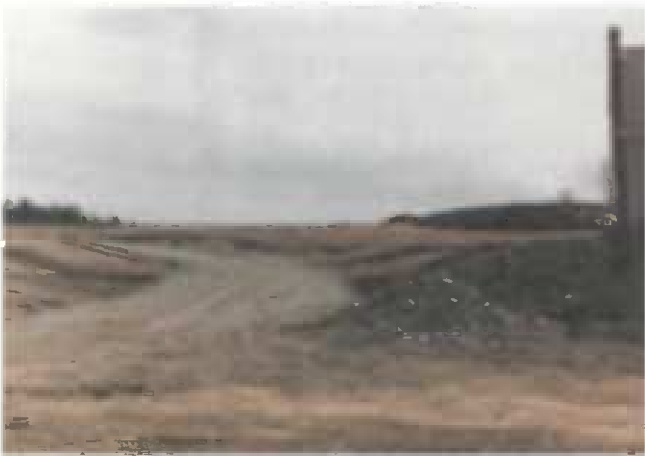
Figures B-6 and B-7: The same site, viewed from opposite directions, shows a long, steep slope mulched to prevent sheet and rill erosion.
