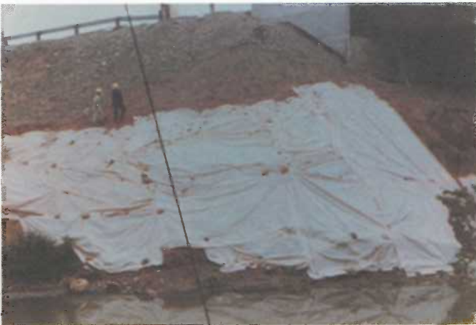
Geotextile used prior to riprap placement.
