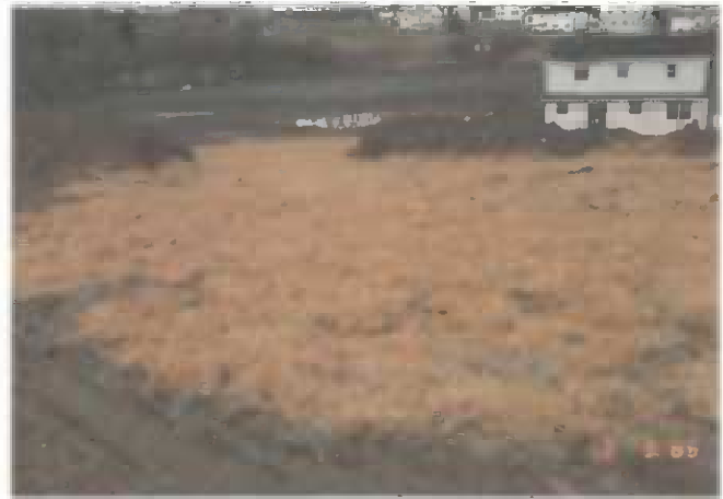
Figures B-6 and B-7: The same site, viewed from opposite directions, shows a long, steep slope mulched to prevent sheet and rill erosion.
