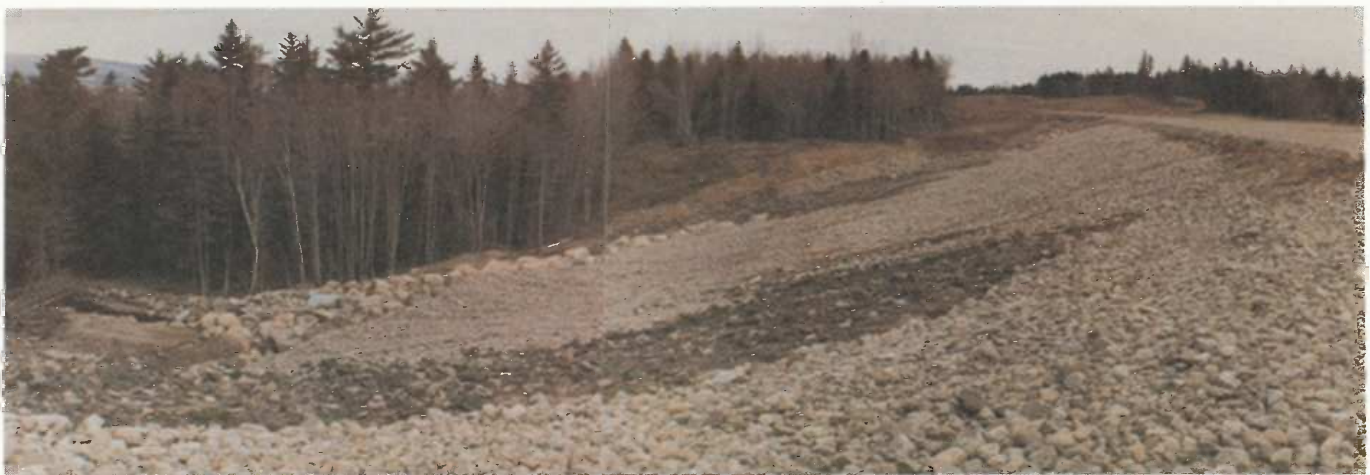
Riprap used on steep embankment.
