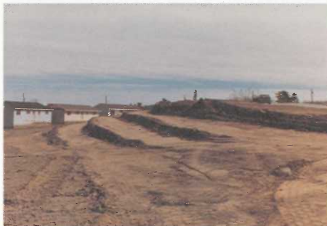
Grading of terraces in a subdivision.
