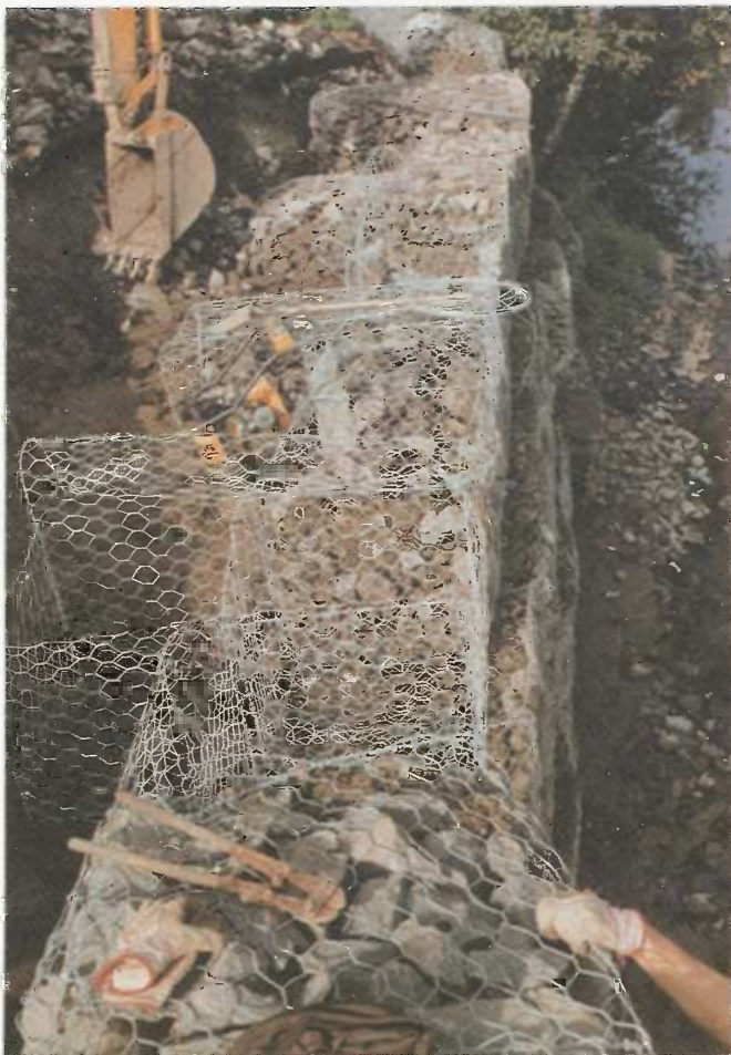
Filling the gabion baskets with stone. Note that each successive layer is stepped back slightly.
