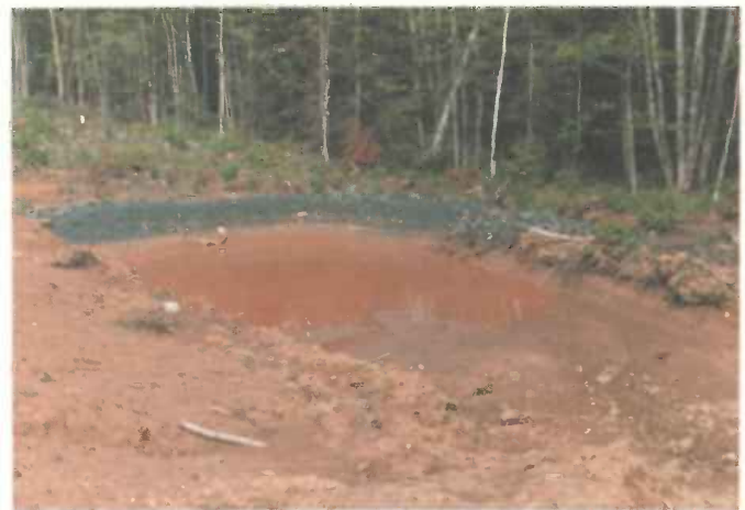
Temporary siltation ponds have a life span of a few months to a few years and provide much more storage than expedient ones.
