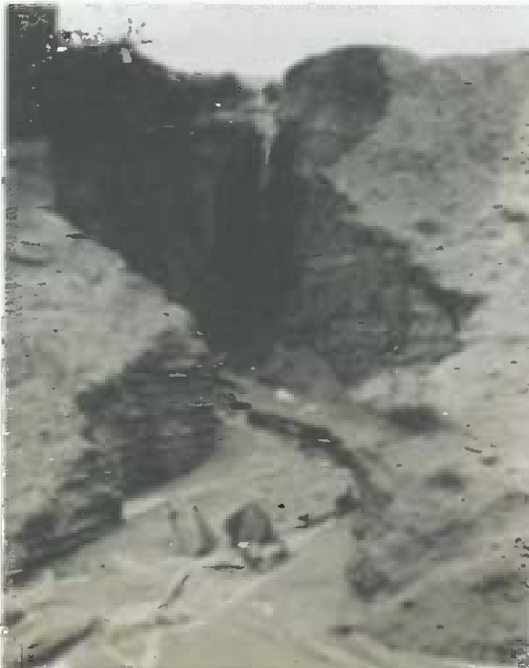
Figure B-3: Sheet and rill erosion occurring on an exposed highway embankment quickly filling in the drainage ditch with sediment.
