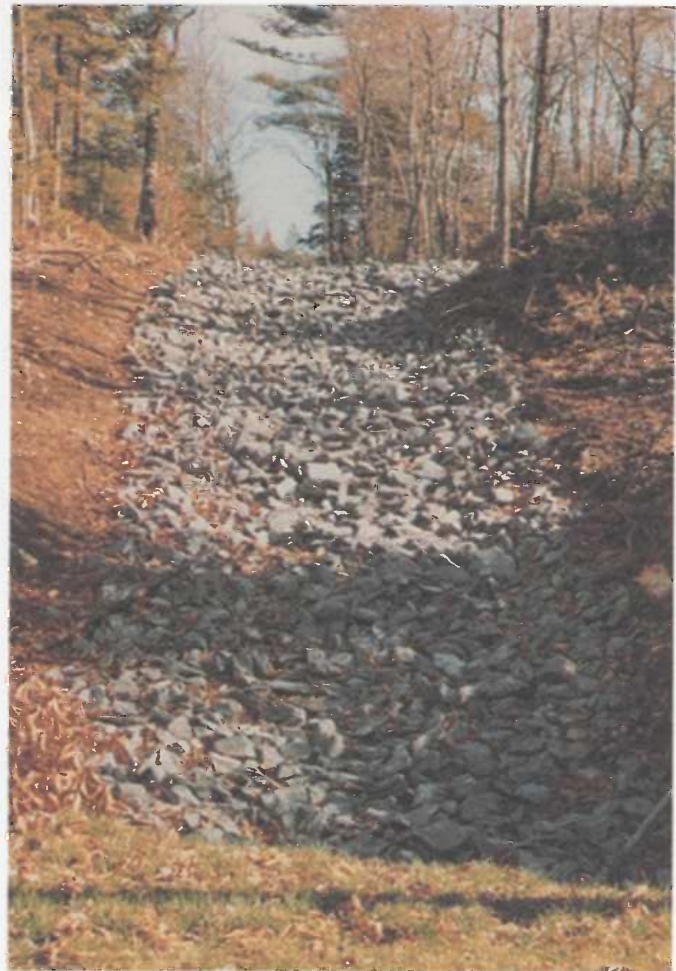
After: a stable storm drainage easement.
