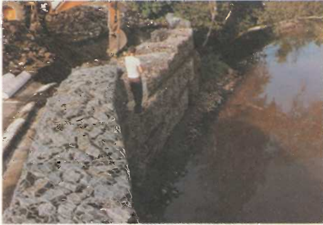
Filling the gabion baskets with stone. Note that each successive layer is stepped back slightly.
