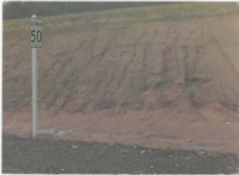
Figure B-3: Sheet and rill erosion occurring on an exposed highway embankment quickly filling in the drainage ditch with sediment.
