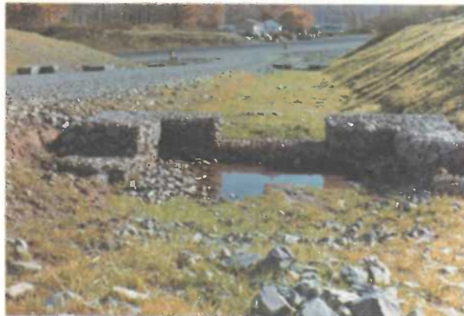
A properly installed series of gabion check dams. Note also the effectiveness of hydroseeding and lining the ditch with rock to achieve maximum erosion control.
