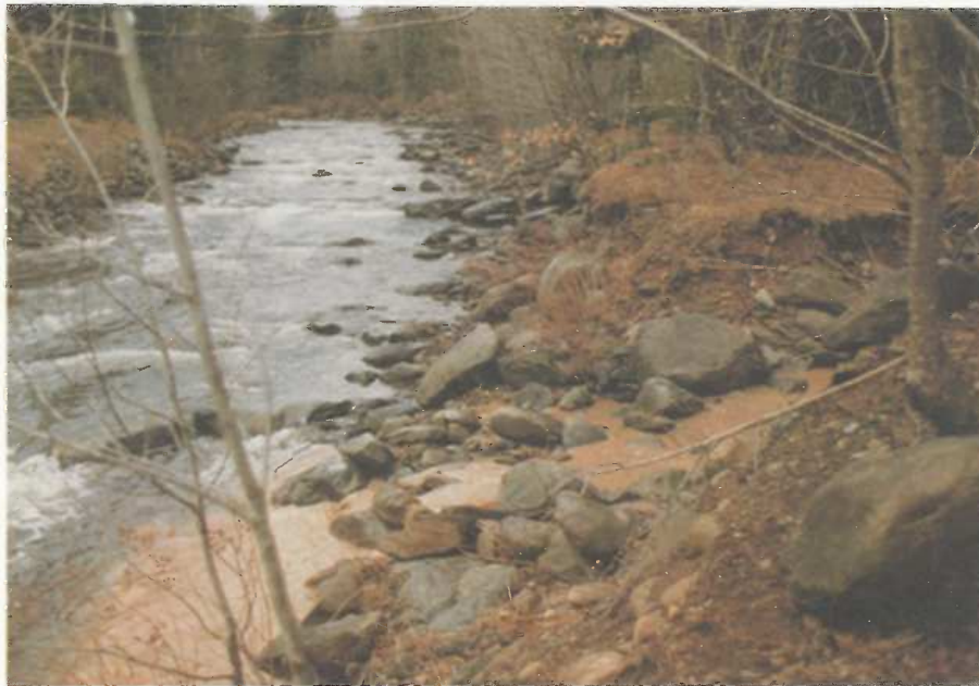
Figure 1: Sediment-laden water flowing into a river from a construction site during a heavy rainfall.
