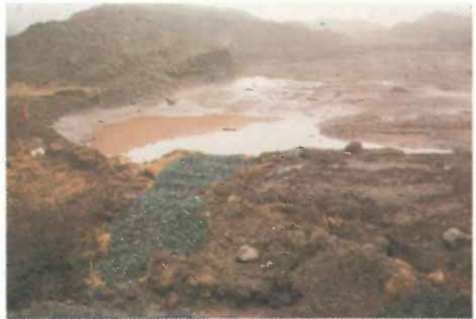
Expedient siltation ponds should be designed for a few days' use and should provide for a small amount of storage. They can quickly be constructed with a bulldozer or backhoe.
